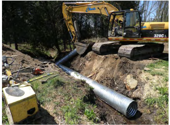
Culvert repair
