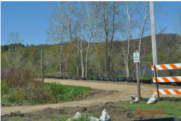
Prepared for repaving
