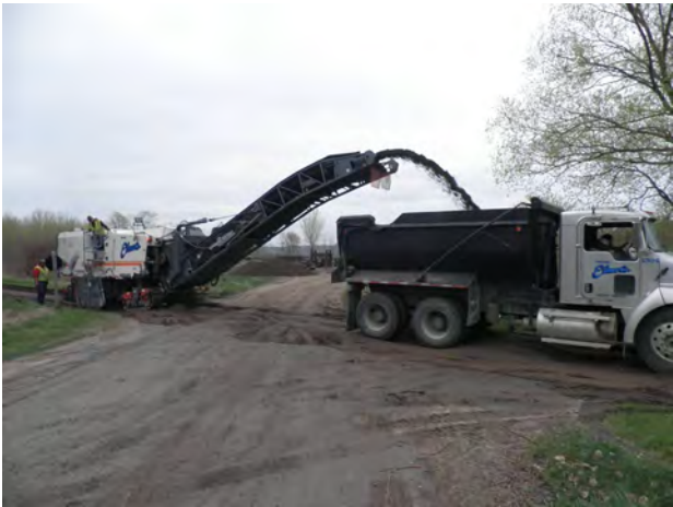
Team Elmer's grinding old asphalt
